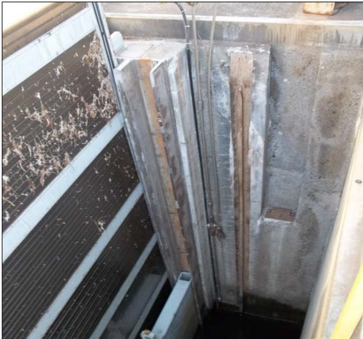
Figure 4-8. Alternative A3 – Modify VBS Perforated Plates
